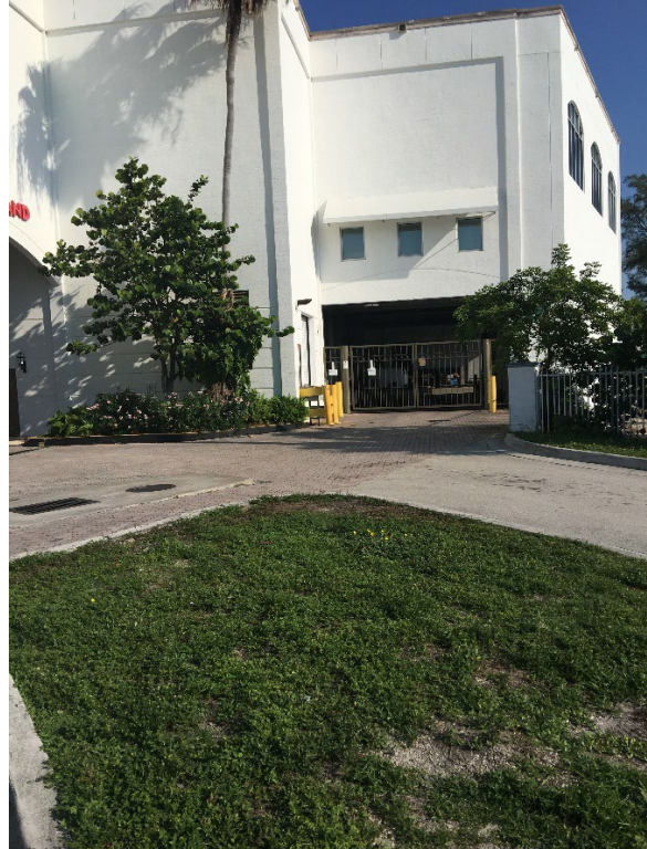
Loading Dock Entrance
